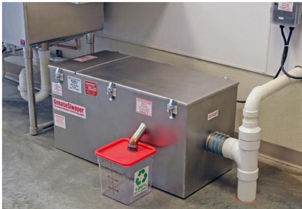
6. Figure 6 – GRD- Gravity Removal Device
