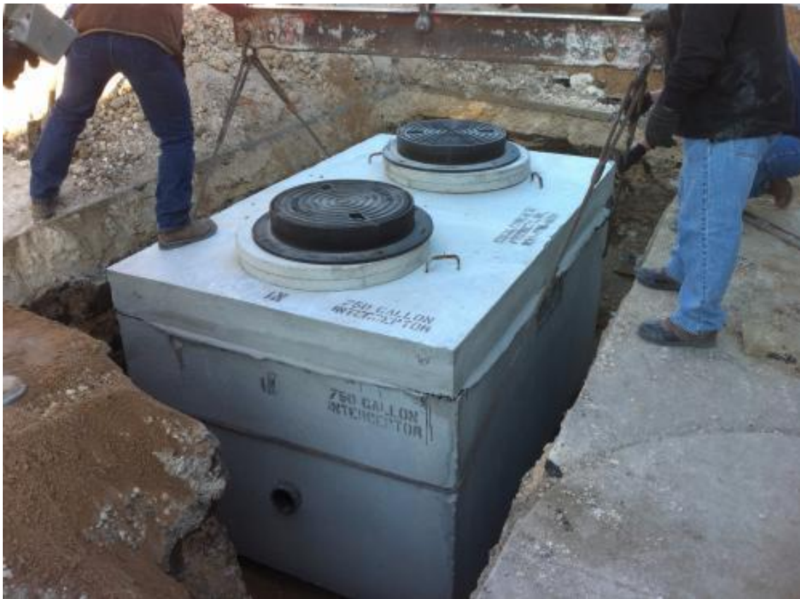
4. Figure 4 – Grease Interceptor
